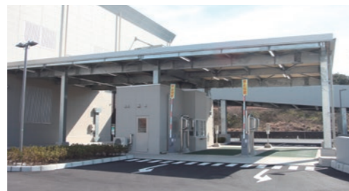
計量棟 Weighing building
